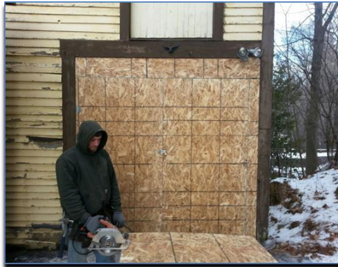
Boarding-up and Securing 1158 Main Street January 2015
