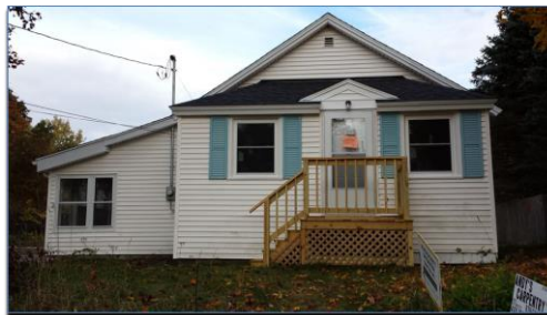
Renovations Completed at 112 Harvard Avenue, Athol
