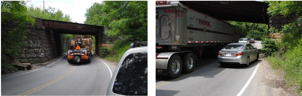
Figure 4.5-1: Narrow Rd & Dangerous S-shaped Horizontal Curve at Rt 31 RR Bridge
