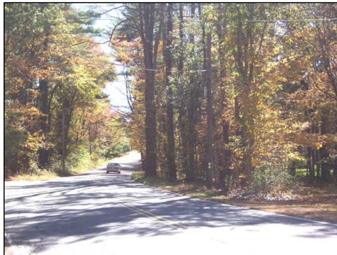
Vegetation Opposite of Beaman Road on Horizontal Curve that Inhibits the Ability of a Driver to View the Roadway Ahead.
