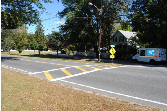
Crosswalks and signage along Route 117 – No curb cuts or direct connection with sidewalk
