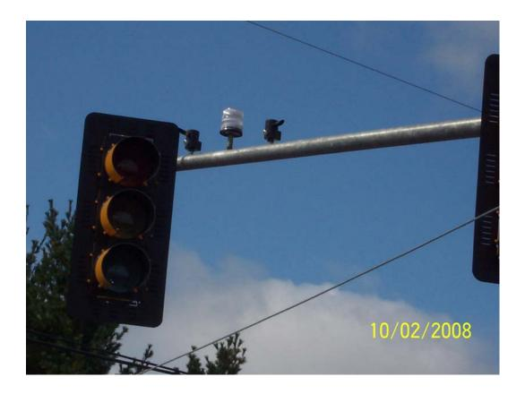
Shown above is a preemption control device located at a newly installed light at the intersection of Rte. 12 and Nichols St. on the Fitchburg/Leominster city line. From left to right are the traffic signal; the notifier; and the preemption sensor.
