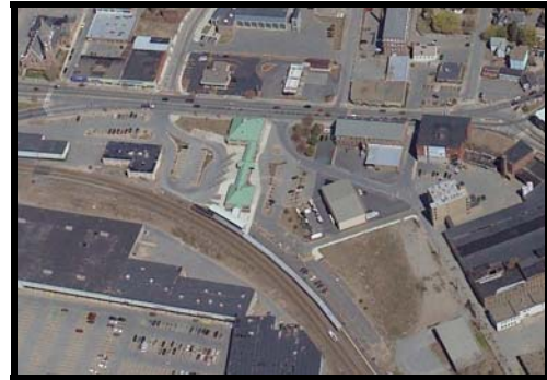
The removal of Caron's Flea Market and Availability of the Summer Street Fire Station and Harper's Furniture Helped Micon Products, Inc. Expand Operations and Grow this Key Manufacturing Business Onto Main Street In Moran Square
