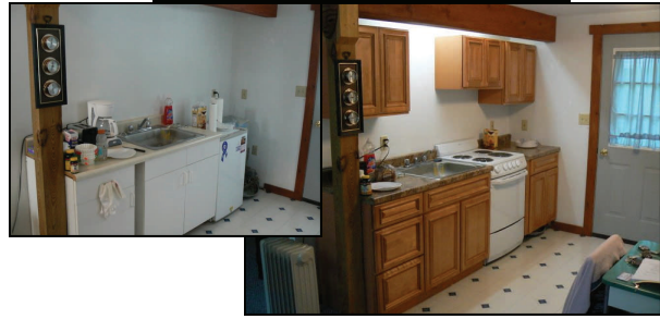
Before/After kitchen rehab
